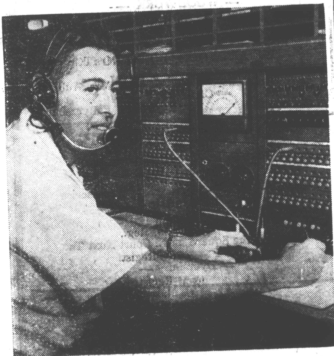
Guided by electronic "eyes and ears", this test deskman spots line troubles at once and gets repairmen there quickly, often before service is actually interrupted.
